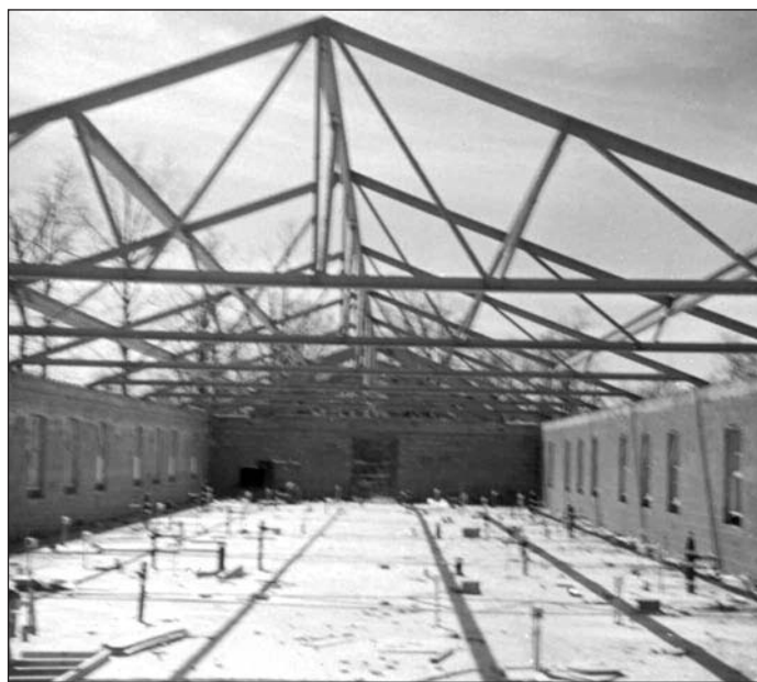
Construction photo of the original Men's Wing
