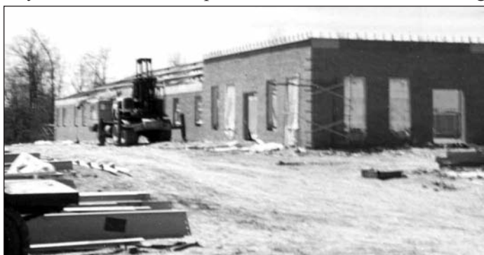
Construction photo of the Day Room
