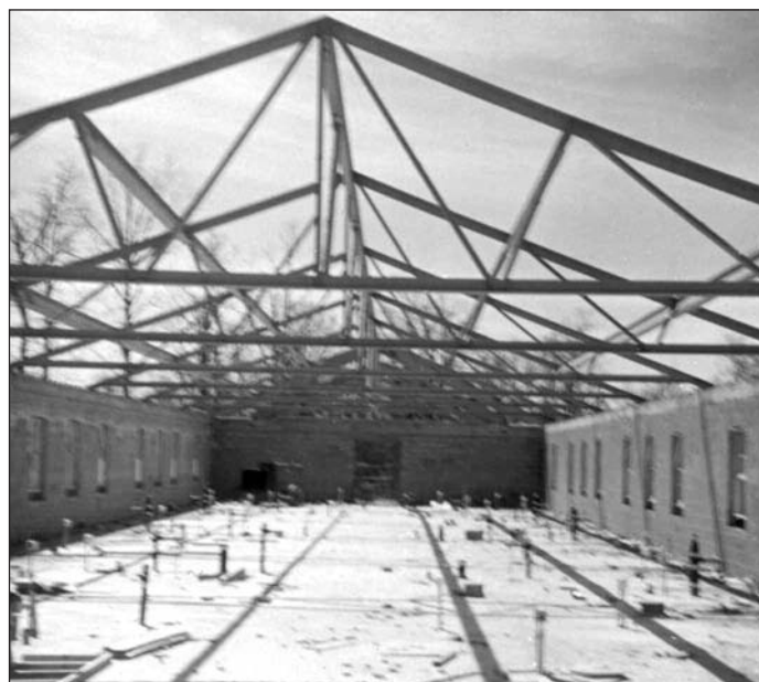
Construction photo of the original Men's Wing
