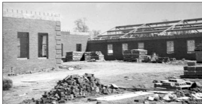
Construction photo of the Rear of Cafeteria
