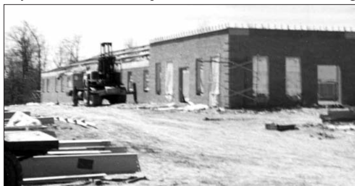
Construction photo of the Day Room
