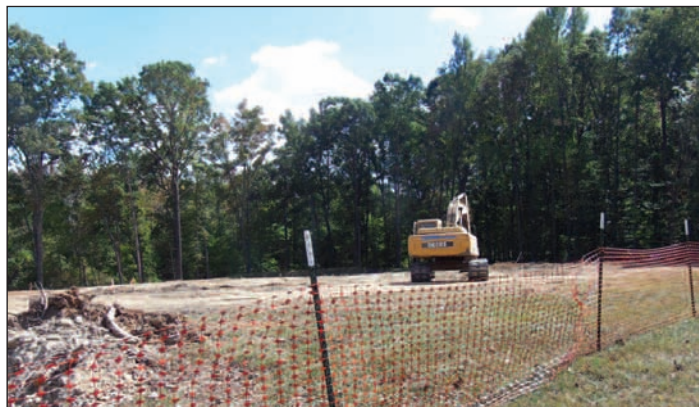
Site prep underway for construction of the Men's Extended Treatment Lodge
