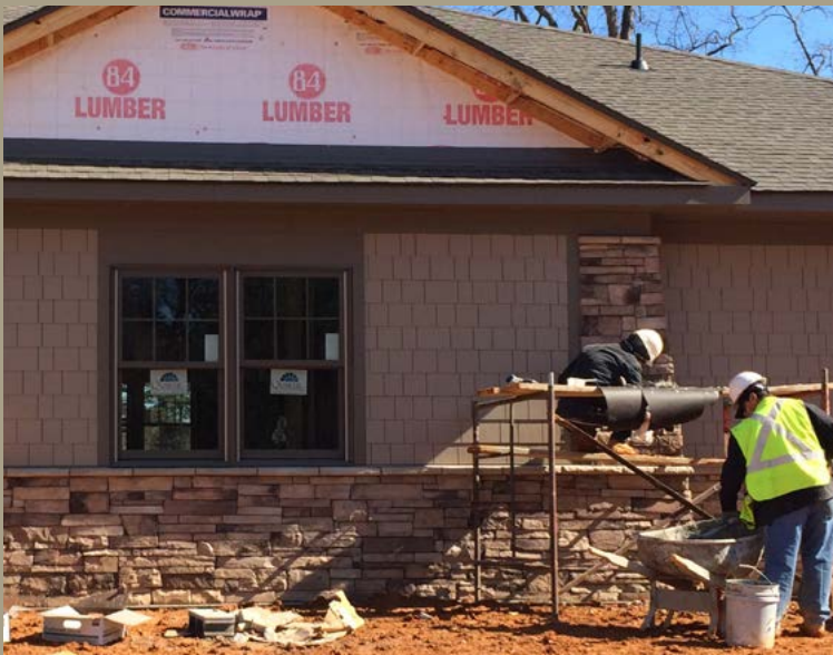
exterior: workers construct stone columns on the outside of the building
