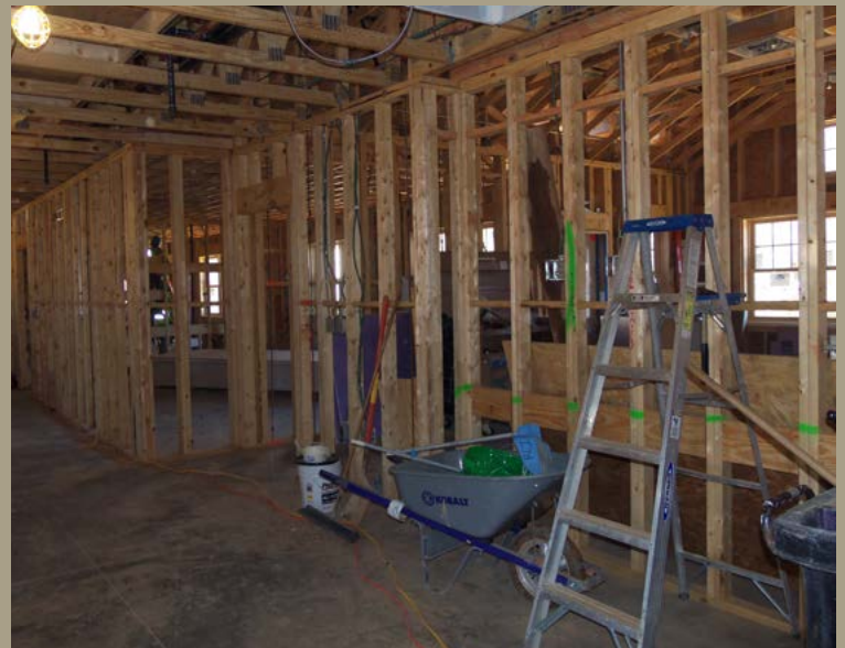
interior: framing and roughing-in of the interior spaces
