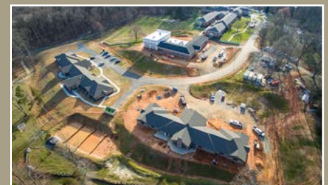
New construction slated to be completed in May.
